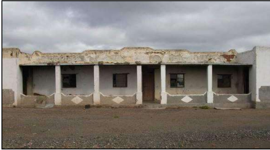
Plate 9: The farmhouse of Kat Doorn Kuil retains considerable heritage value as a typical Karoo style flat roofed structure.
