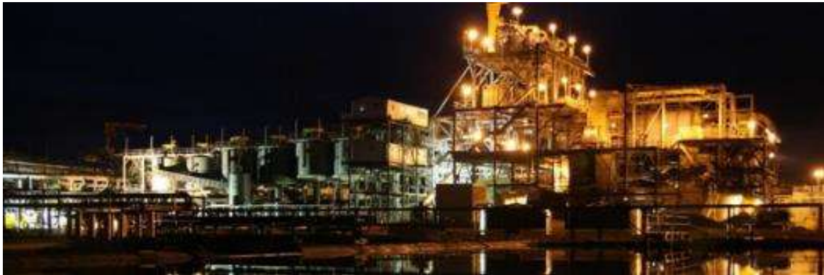
Figure 4: Example of Processing Plant as seen at night
