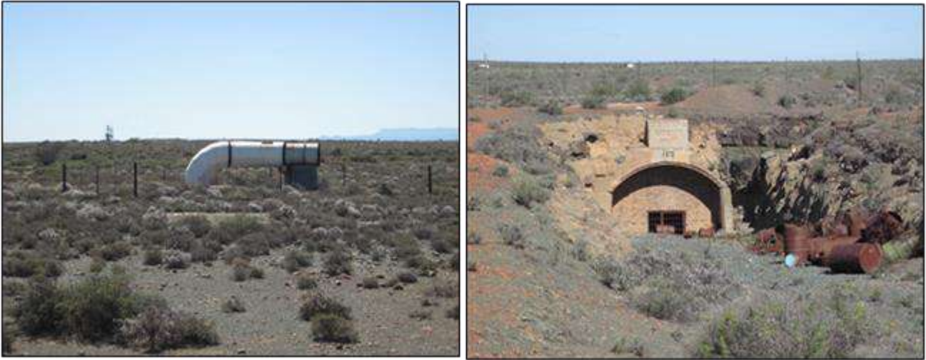
Plate 3 & Plate 4: The existing mining infrastructure on Ryst Kuil Main dating to 1978.
