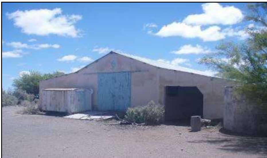
Plate 8: The view of the shed on Ryst Kuil.
