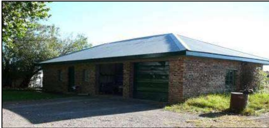
Plate 62: The garage and shed at Water Gift.
