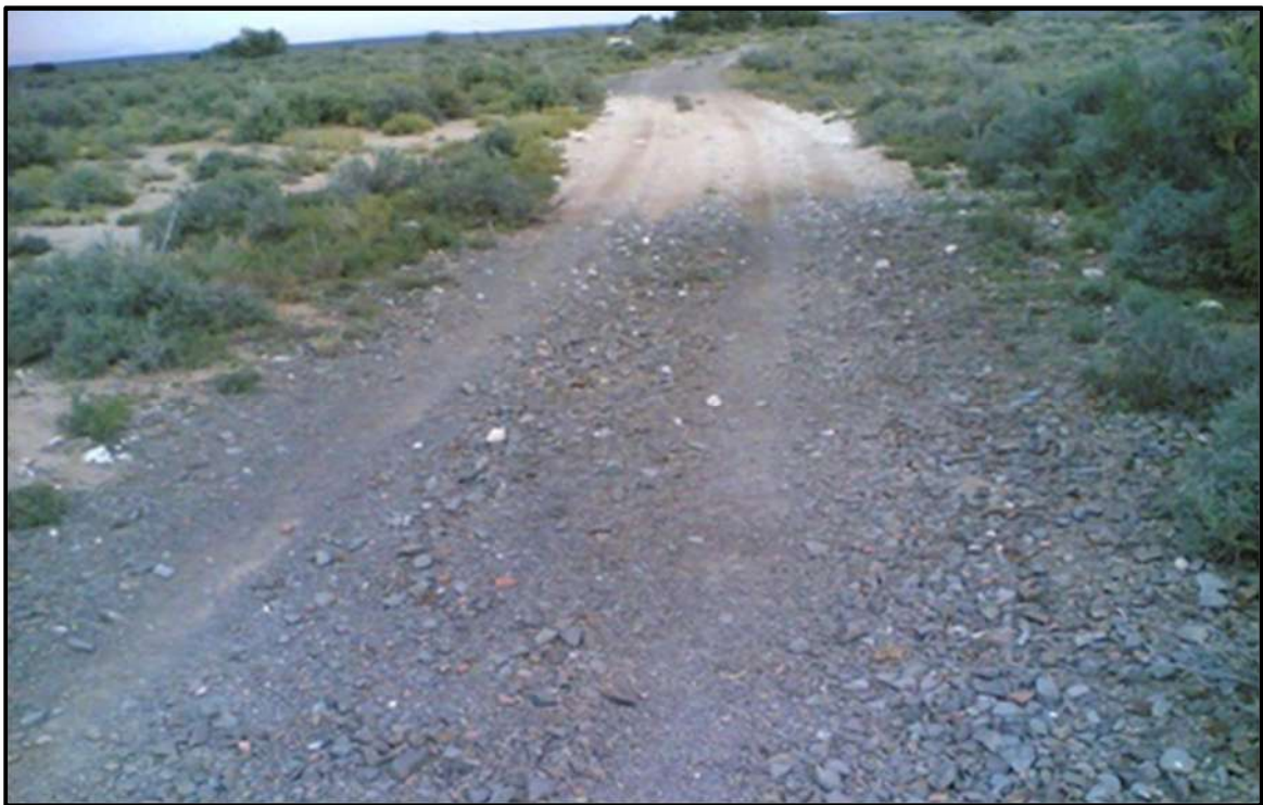
Figure 2-5: Radioactive uranium ore used to fill potholes on a farm road near at Ryst Kuil
