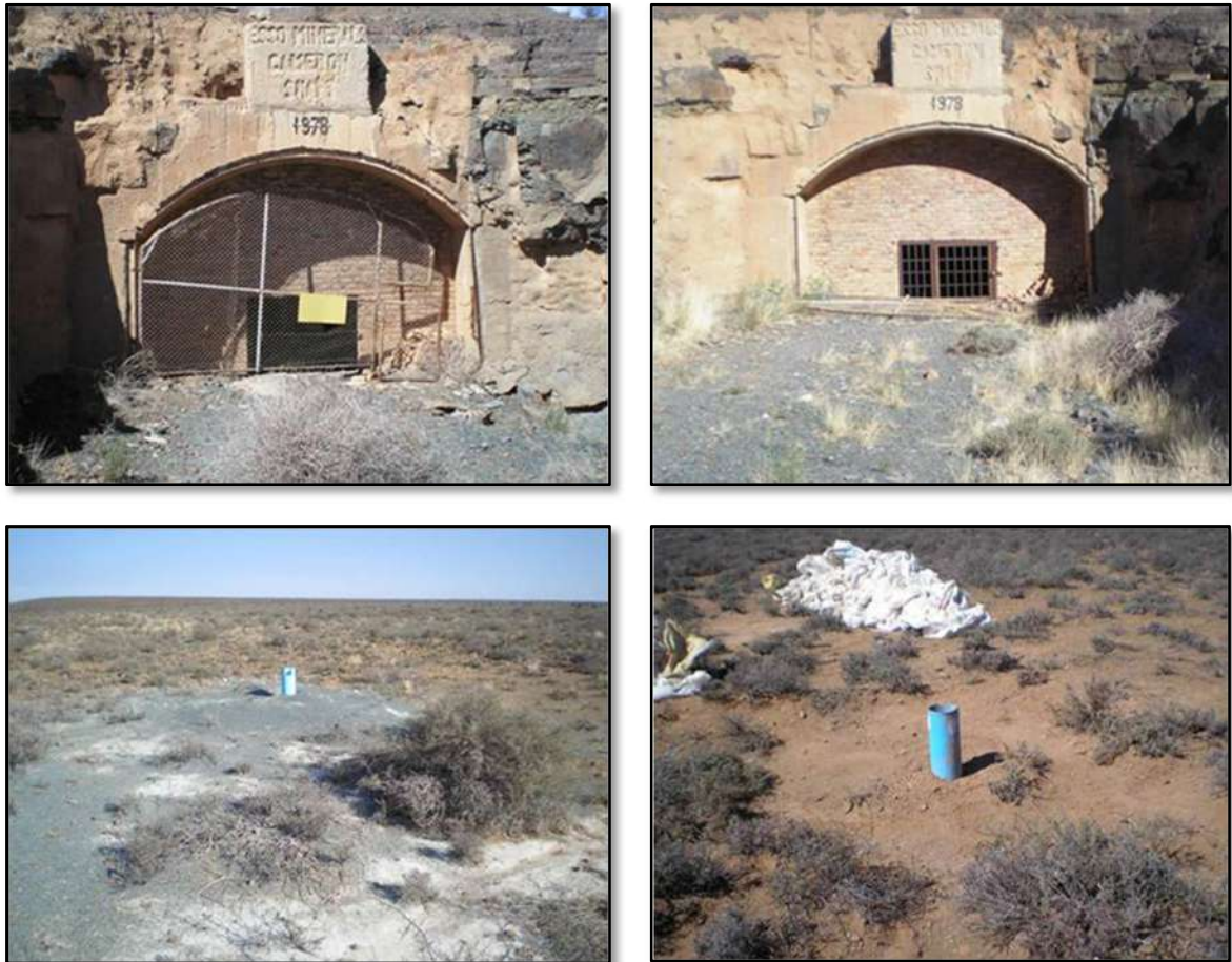
Figure 2-6: Before and after illustrations of the Cameron shaft entrance and a drill sites
