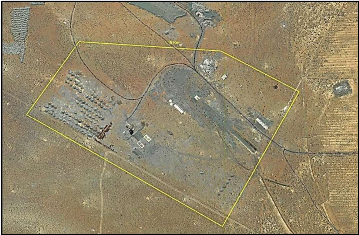
Figure 2-4: The main contaminated area where ore storage access to underground mine area (Cameron shaft) and the crushing plant were located
